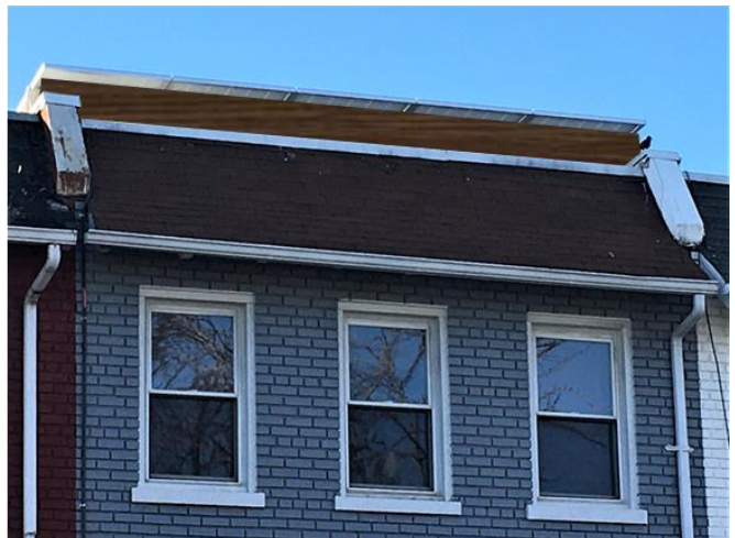
View with solar panel structure screened - wood
